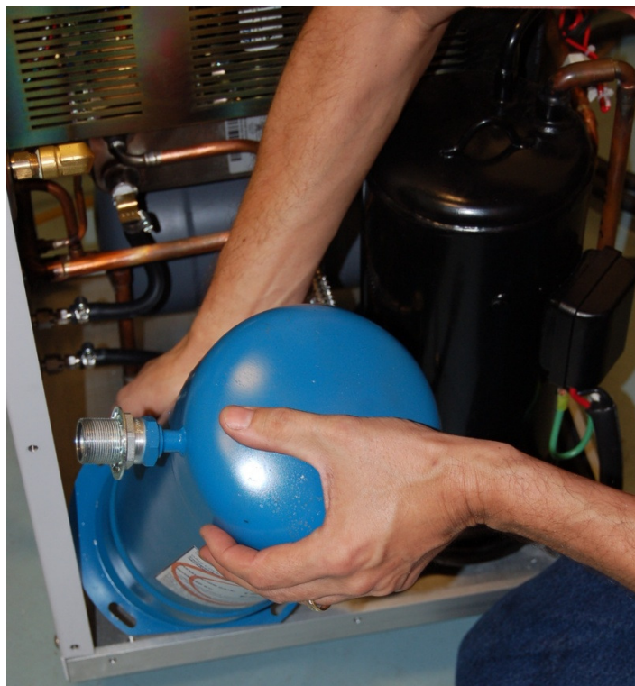
Figure 10 – Adsorber Removal
