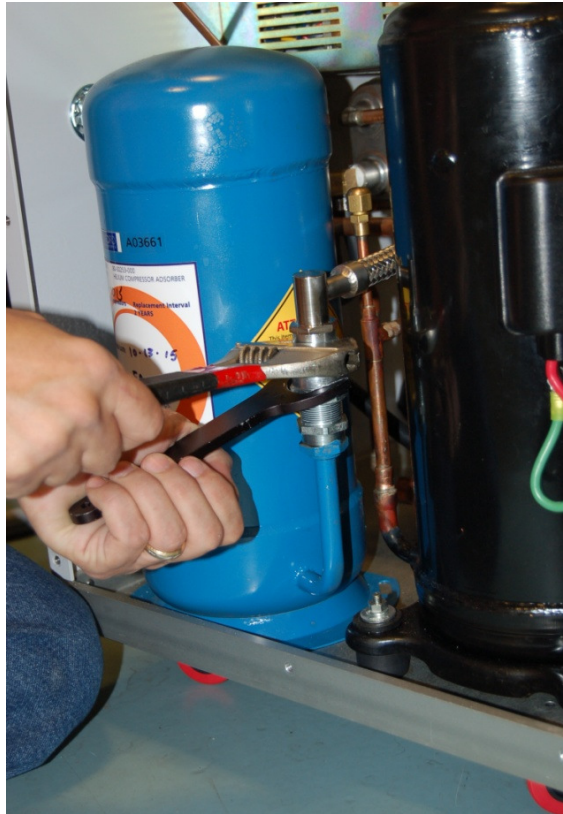
Figure 7 – Adsorber Aeroquip OMS Supply Line Removal
