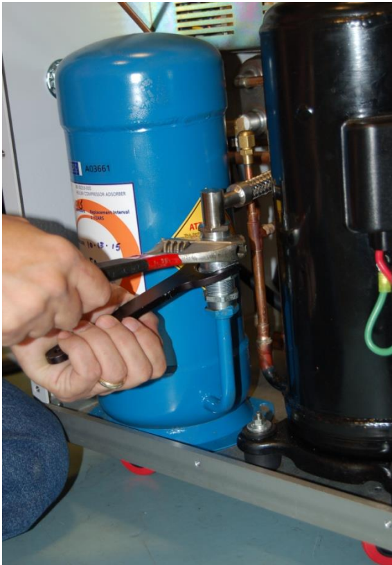
Figure 7 – Adsorber Aeroquip OMS Supply Line Removal
